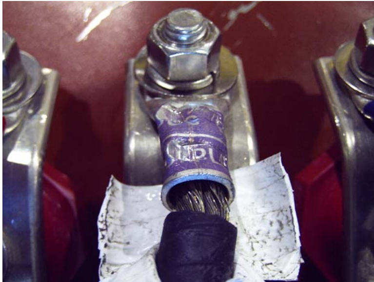
Figure 3 – Incorrect motor termination. 4/0 gauge (purple) crimp lug on 2/0 gauge wire, not crimped and soldered or crimped utilizing a hexagonal style crimping die
