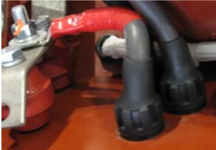
Figure 6 – Sealing gland eliminates air gap around motor leads entering junction box
