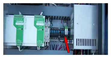
This breaker MUST be opened to prevent damage to the winch valve manual actuator linkage.
