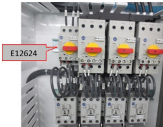
Figure 1: TD Lube Pump Motor Circuit Breaker
