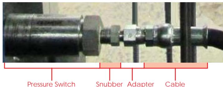
Figure 2: Add snubber between pressure switch and connection adapter as shown
