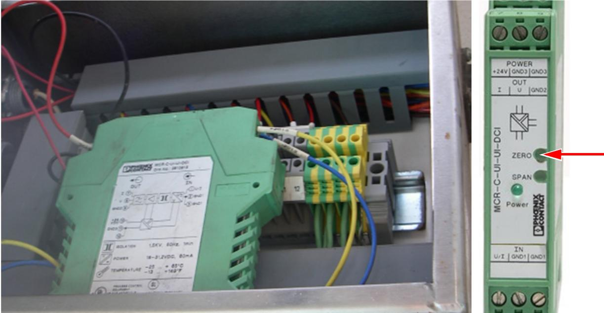
Figure 1: Signal Conditioning Card
