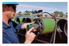
Installation is fast and easy with a simple handheld hydraulically actuated tool. Rings can be installed in the field, pipe yard, and/or pipe mill.
